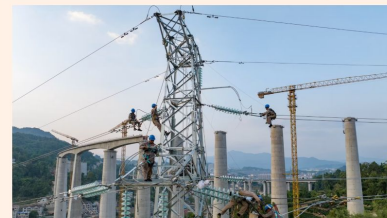
Chinese employees work on an electricity pylon. Electricity prices explain almost 60% of the levelised cost gap of building a data centre in China compared with the UK © CPOTQ/Reuters
